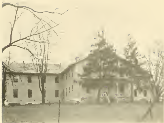
DELAWARE COUNTY INFIRMARY, BROWN TOWNSHIP
